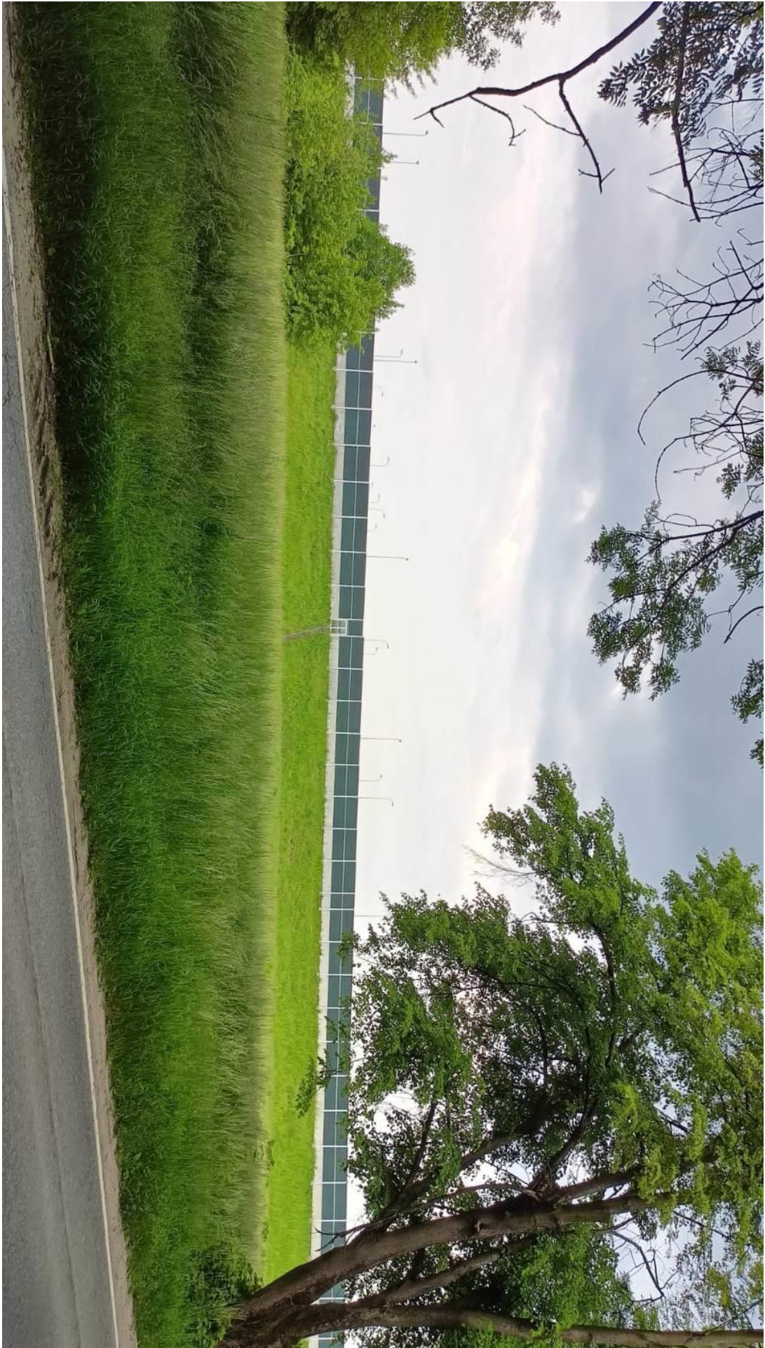
Fence around a highway – protects the environment from the noise
